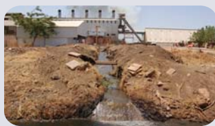
Industrial waste water disinfection
